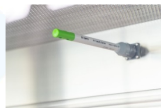
Internal air velocity probe for monitoring.
